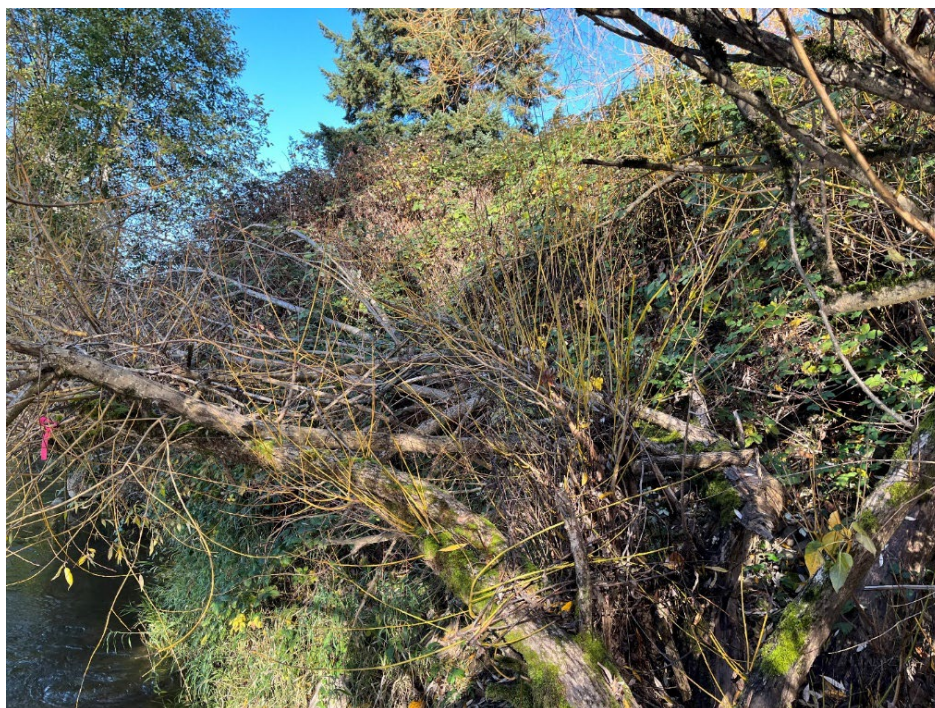
Photo A-12. This photo highlights the existing vegetation of the Horseshoe Bend Levee and the steepness of the riverward levee slope.
